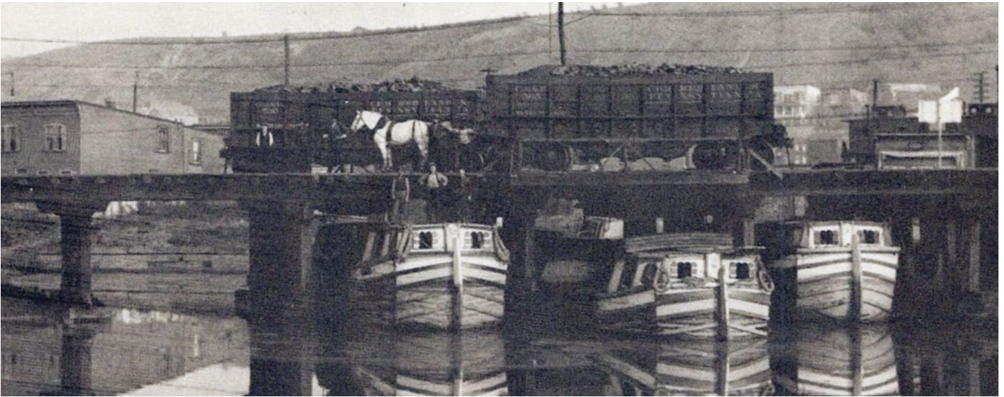
The canal reached Cumberland, Maryland, in 1850, realizing the vision of shipping coal eastward by boat. Soon, coal was brought to the port by rail and loaded into boats—10 tons per car and 12 carloads per boat. Photo courtesy National Park Service
