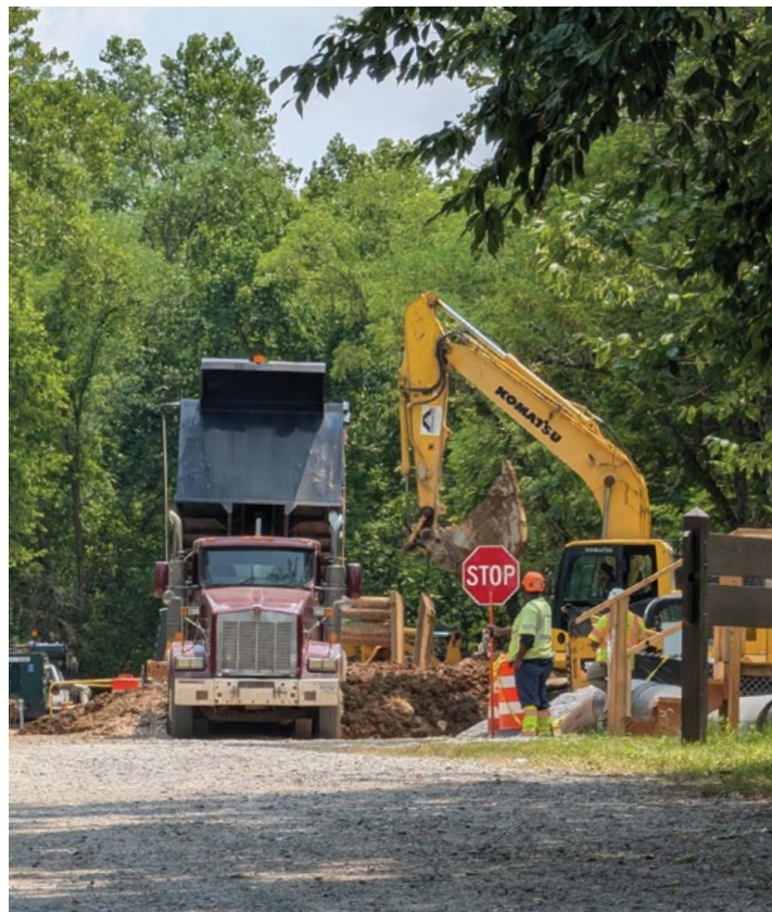
(Left) Bypass pipeline at Pennyfield (Lock 22 near Potomac, MD). This large pipe runs along the berm side of the canal. (Right) Construction of the bypass pipeline at Pennyfield. Photos by Jon Wolz
