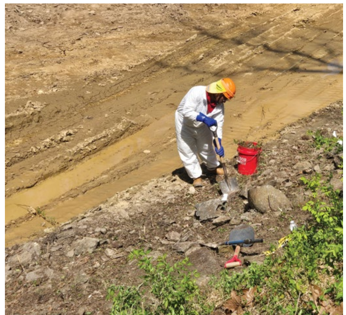
(Opposite, top) Temporary dam bridge holding fresh Potomac River water to be used to “flush” the canal at Lock 14. (Opposite, bottom) Reinforced access point for work equipment between Locks 11 and 12. (This page) Worker removing waste product near Lock 12. Photos by Allyson Miller
