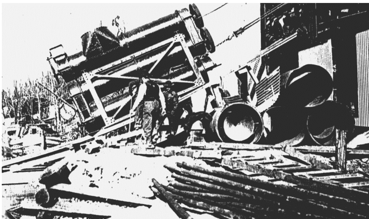
44. Using an inclined plane and winches to get the hydrator in place Courtesy Washington County Public Library
