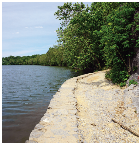
Stone causeway partially scoured by flood waters
