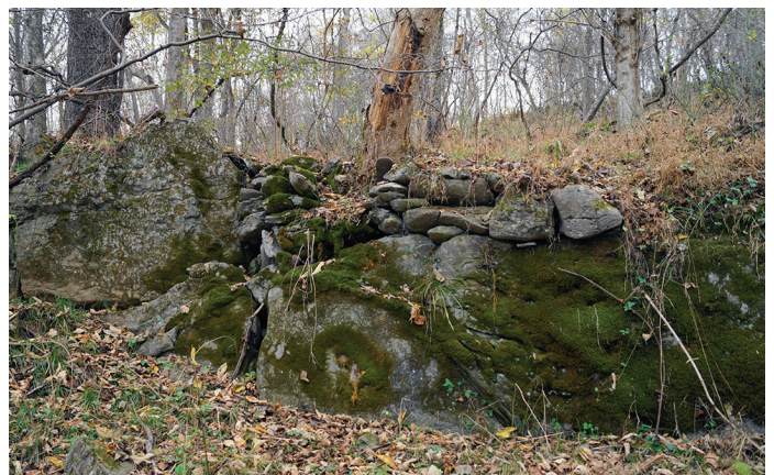
Improvisation and use of the environment are often overlooked in examining the lives of our predecessors. I really like this wall; a natural outcropping was neatly added to the fieldstone to create a higher wall.
