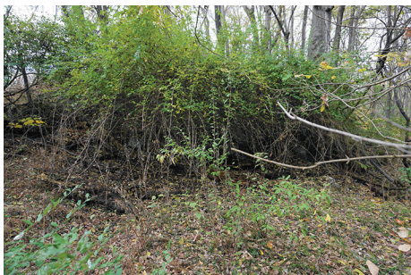
To the west of the Denton Jacques warehouse, after fighting through the thorns and weeds, you can find the foundation remains of the Flory House and garage built into the river-facing hill.
