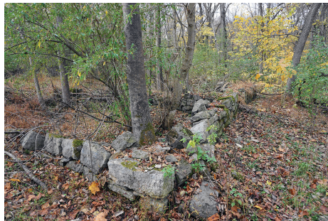
Foundation remains of the Fernsner House located just to the east of Lock House 49.
