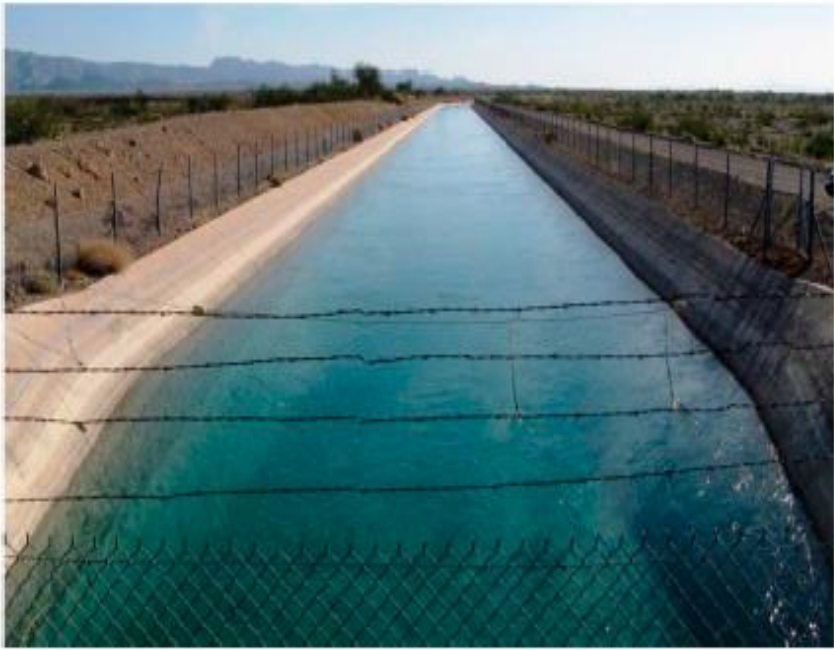
Figure 2. Canal in the Mojave Desert of California showing wildlife-proof protective fencing along the edges. Photo taken from a road across the canal.
