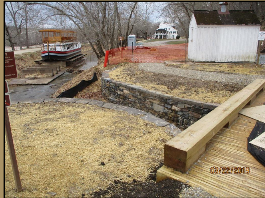
Lock #19 Canal Wall Repair
