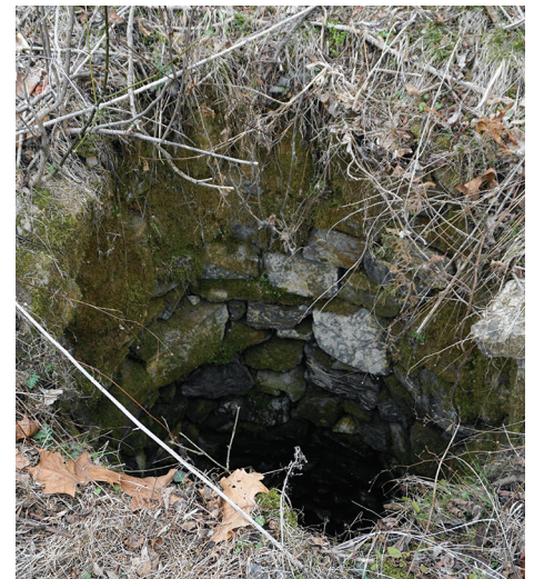
Open stone lined well, about four feet in diameter
