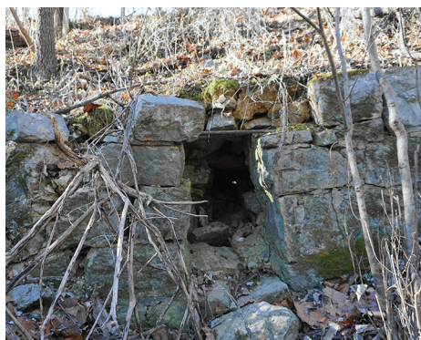
Limestone box culvert under the railroad grade
