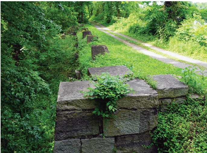
Formal overflow/waste weir at Mile 113.48
