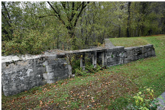
Above – A waste weir is built into the aqueduct structure on the berm side
