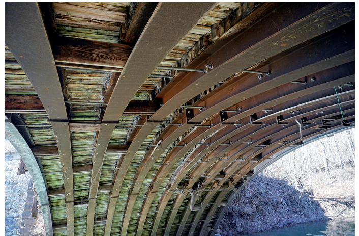
Above – Some of the intricate structural steel support structure under the aqueduct's single arch
