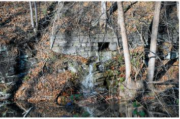
A box culvert under the abandoned Western Maryland Railway right-of-way in the Town Creek area. It drains into the C&O Canal.
