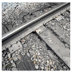
A loose sleeper. When the ground is wet and a train passes over, a slurry of coal mud washes out.
