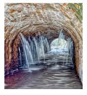
Culvert 185, at Mile 126.42, is a 10-foot span sandstone culvert with a 5-foot rise. Also called Johnson's Culvert, it was built in 1836-1837. The stream is moderately active. When the prism above the culvert is watered the barrel leaks through numerous holes, creating a car wash effect. Upper - berm arch; side – barrel; lower – towpath arch. – Photos by Steven Dean
