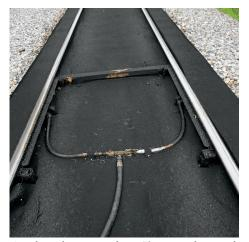
A mechanical monitoring device. The area on the ties and under the felt is soaked with petroleum grease.
