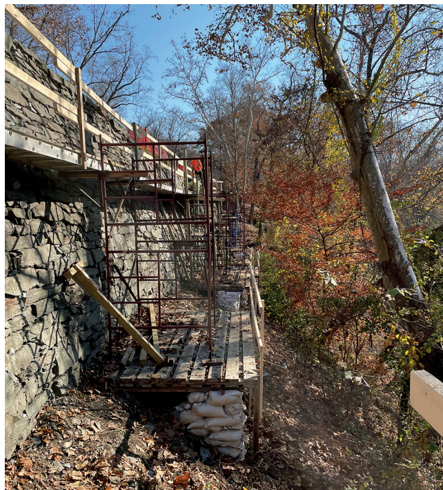
Top: A pedestrian bypass detour around the project site.
